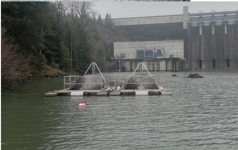
**Figure H-12. Lookout Dam Tailrace – Powerhouse Channel in the old orientation where one trap was staggered behind the other (top) and in the new orientation side by side (bottom).**
